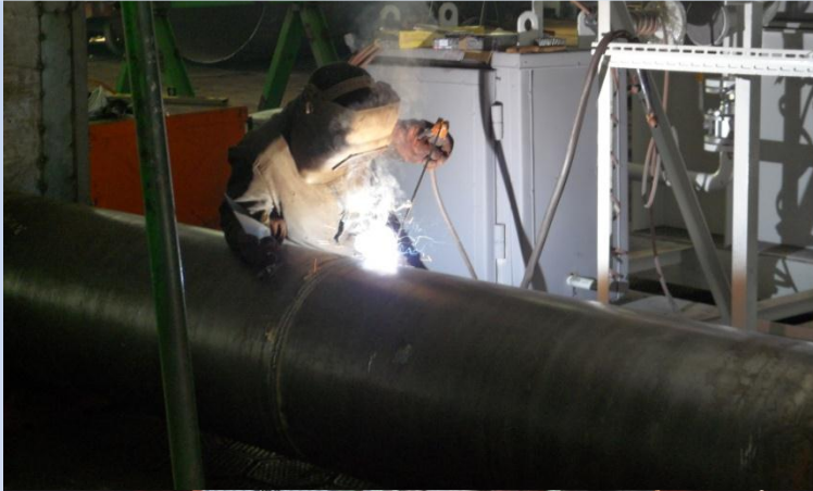
Manual arc welding
