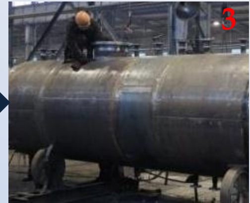
Assembly and welding of bulks and neck seal
