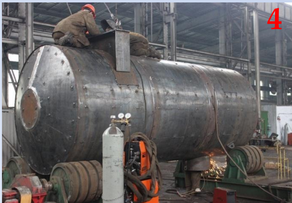
Welding of holders
