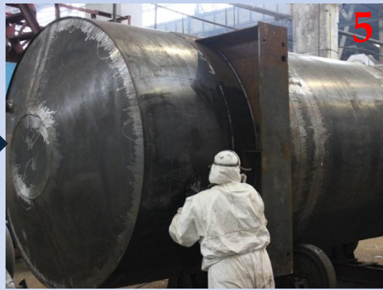
Preparation for painting
